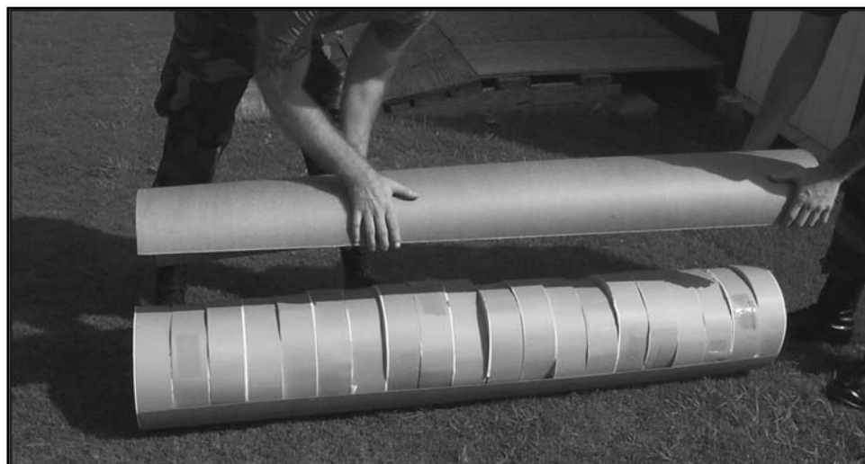
Figure D-15. Cardboard tube placement
